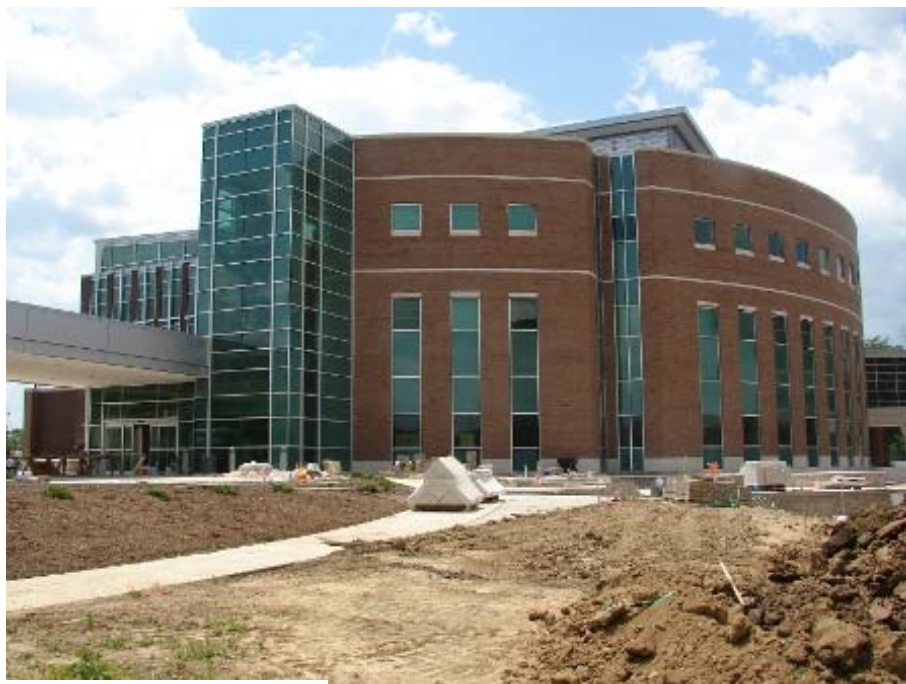
Progress on SCCI building 6/18/08
